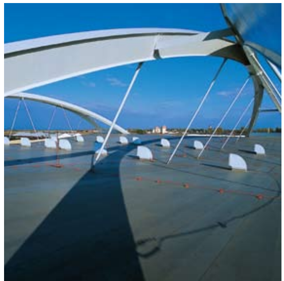
Transport station (Czech Republic)
